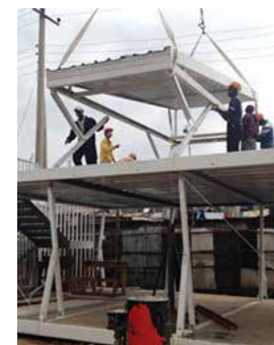
Hoisting of the pre-fabricated panels in progress.
