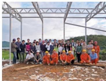
Architects and university students took part in the construction of New Bud Study Hall
