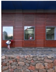
With a simple timber-trellis cladding design, this modern building blends in with the rural ambiance of the village
