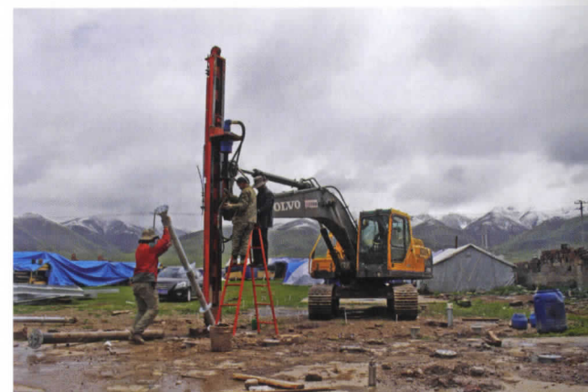
Figure 9 Installation of Ground Screw
