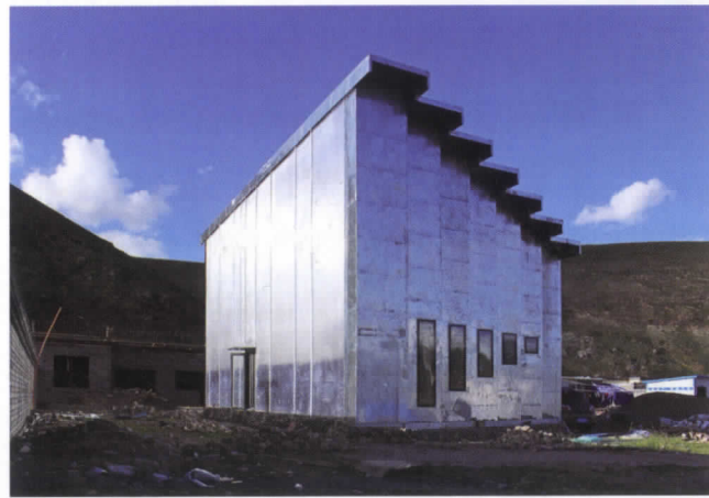
Figure 7 South-west view of New Lawuga School
