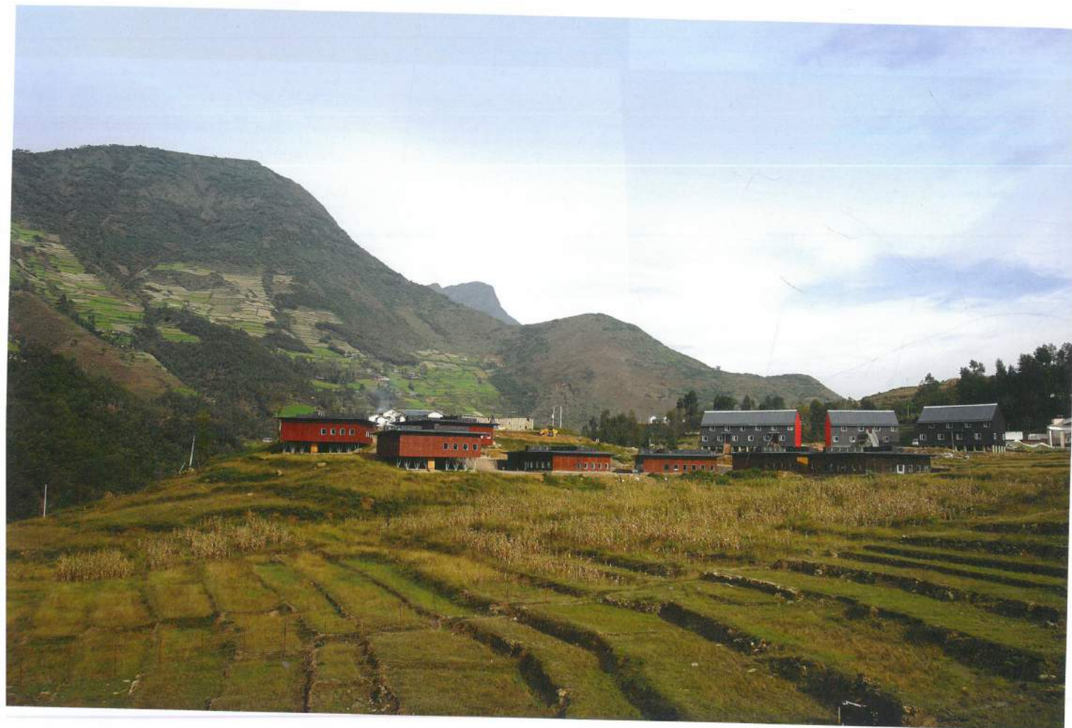
眺望美姑红丝带民生爱心学校教室与宿舍群，落在坡基之上的红色与灰色量体漂浮于坡地。 Classrooms and dormitory complex in Meigu Charity School, with red and grey volumes elevated above the slope.
